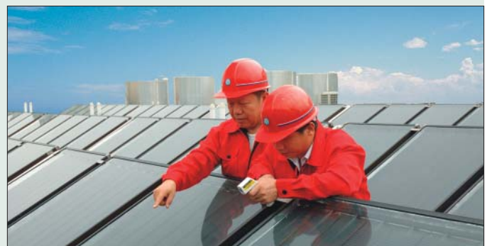
Huisheng's solar-powered water heating system
