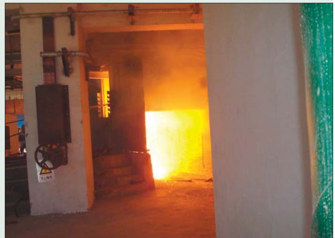
Ruichi's cogeneration smelting furnace
