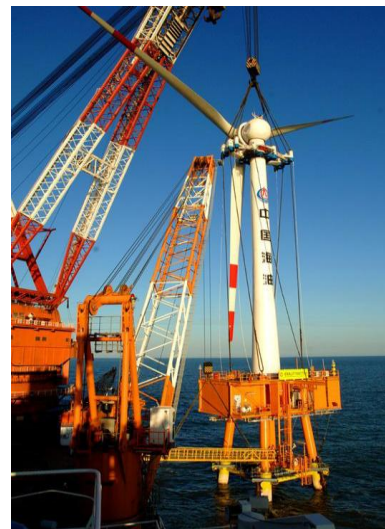
Figure 6: Bohai turbine installation
