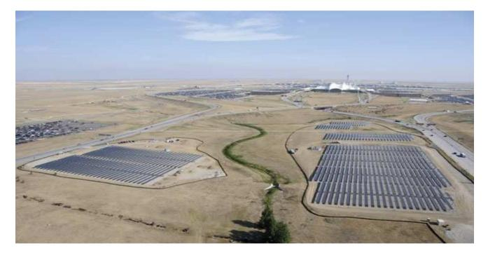
A second, 1.6 MW PV array was brought on-line in March 2010 to provide 100% of power for one of the airport's fuel-storage facility.
