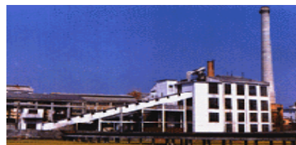
Fig 5-4 65 t/h Bagasse boiler
