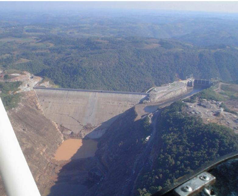
Damage to upstream side of Campos Novos Dam in Brazil after uncontrolled emptying of reservoir. This 880 MW completed project is seeking CDM validation.
